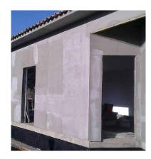
Starting from top to bottom, the high-density BetonNet Glass 360 glass fiber mesh is unrolled (360 gr/m²); the overlap of the nets must be about 10 cm.
