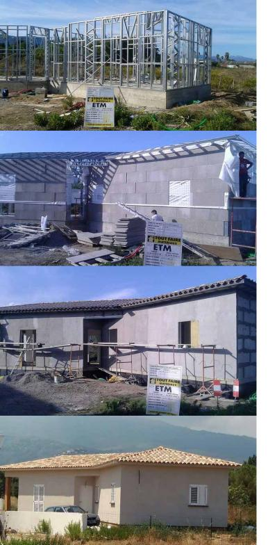
Here on the side we can see the main phases of dry construction of our BetonWood system on a metal frame structure.
