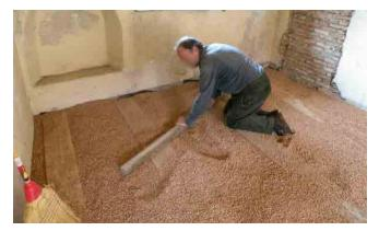
After an appropriate dry trowelling of the granulated cork, the BetonWood cement bonded particle boards can be fixed with screws passing through the supporting substructure.
