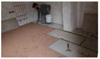
Example of cement bonded particle boards BetonWood TG for renovations, small size: thickness 20 mm, size 1200 x 500 mm, tongue&groove edges.
