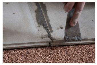
For proper grouting and gluing we use specific products such as BetonElastic, a cement mortar that works both for grouting and gluing, filling the joints between the panels.
