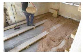
The thicknesses and the sizes of the dry screeds to be used depend a lot on the inter-axis of the load-bearing structure and on the accessibility of the area.
