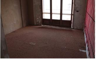
In the case of a totally floating structure on granulated blond cork (as we can see in the figure) we reccomend to install cement bonded particle boards with tongue&groove edges BetonWood TG laid by staggering the joints and screwed on each other, with offset arrangement.
